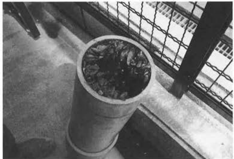
Fig.2 Mytilus galloprovincialis , obstructed inside of service (discharger) pipe.
